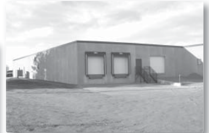
Electro's new building nearing completion.
